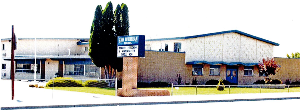
Figure 14 2013 photo of Zion Lutheran School
