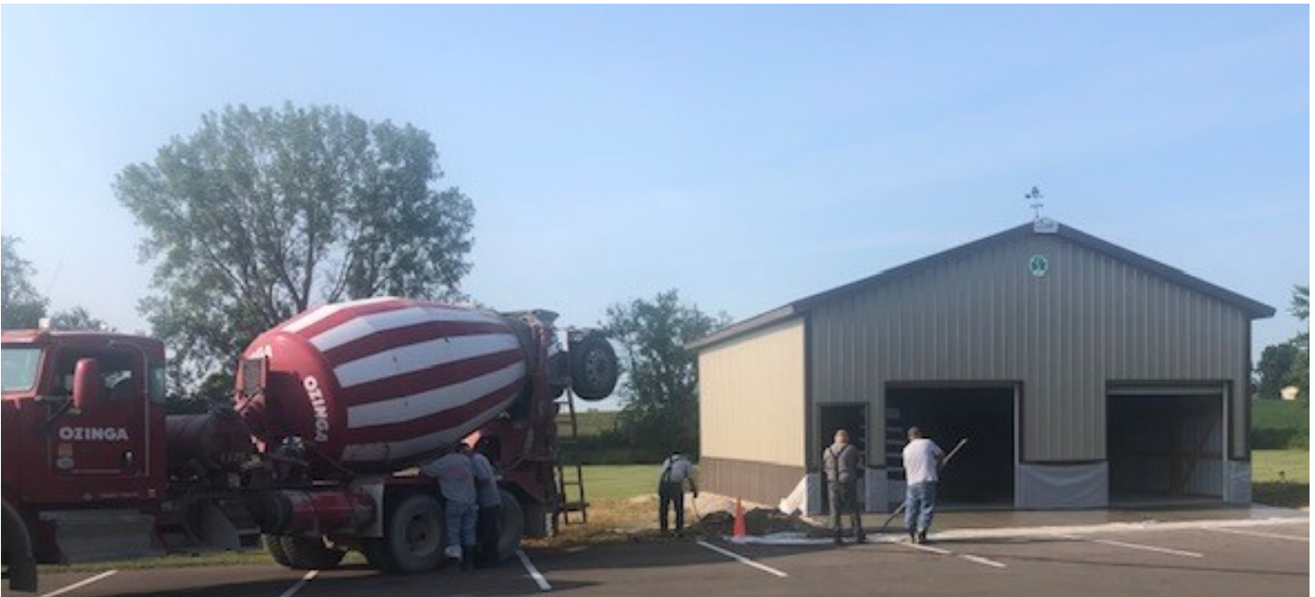
Hard at work finishing the Pole Barn by pouring the apron.
