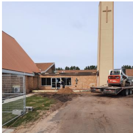
Compacting after the footings were backfilled. It's noisy!
