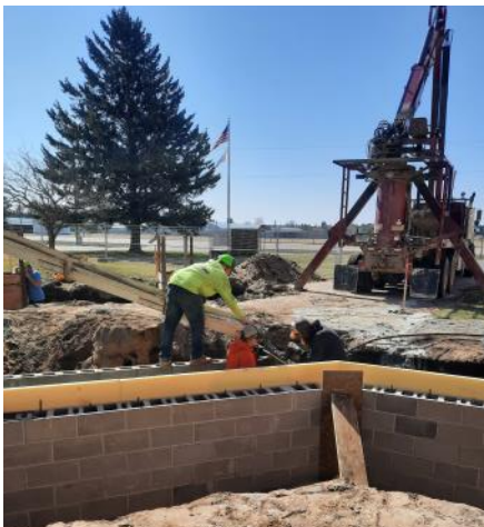
Pouring concrete into footings on one of the nicer days.
