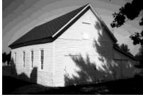
riding mower. You can see here the two new doors in the south (originally east) wall. Because of this adaptation and the cuts that were made in the timbers, this wall was in the worst shape of the four by 2013. But using original tie-beams from the attic, most of which are still in very good condition, we can restore this end to be much like it was at first, with two windows. In the new orientation, this wall will be the east wall—which is what it was originally.
