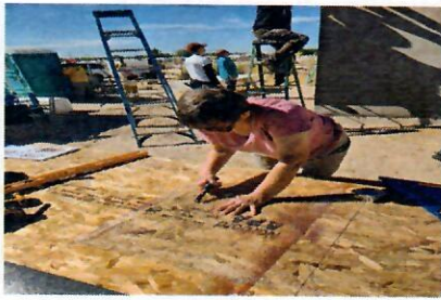
Measure twice, cut once. She's not trying to cut plywood with scissors. She's trimming mesh.
