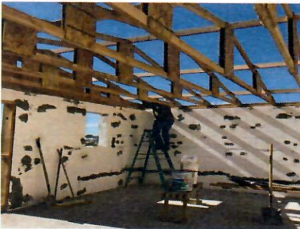
The trusses had been built by a prior group; it was our team's job to get them hoisted up and secured prior to adding the sheathing. Material.
