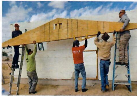
The trusses had been built by a prior group; it was our team's job to get them hoisted up and secured prior to adding the sheathing. Material.
