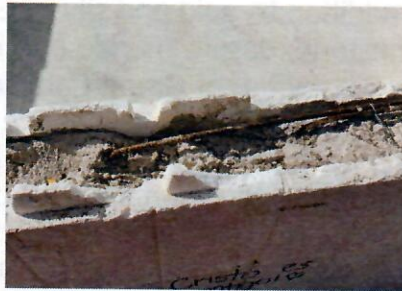
Styrofoam blocks, reinforced with concrete and rebar, are used for the foundation and walls. This results in a stronger, more enduring structure.
