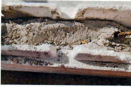
Styrofoam blocks, reinforced with concrete and rebar, are used for the foundation and walls. This results in a stronger, more enduring structure.
