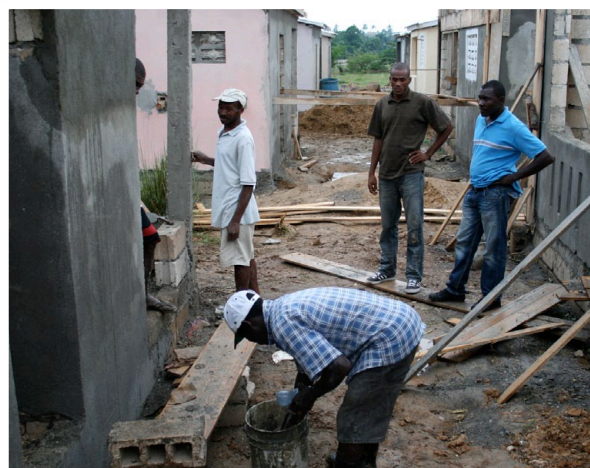
Haitian craftsmen apply a skim coat to cinderblock walls, a common building practice in Haiti. Local workers are employed to strengthen area economies that suffered greatly after the 2010 earthquake.
