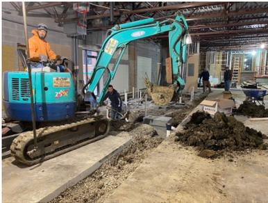
Work continues on our project! Plumbers have been busy laying in the drain lines for all the kitchen and restroom renovations in place so we can pour the new concrete floor before the end of the week.
