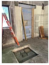
Begin to begin.... After what has seemed like forever we should see construction onsite starting Monday! The bases for the installation of the posts for the new south stairwell have been poured and the steel is supposed to arrive Monday. Once this is complete, we'll be able to start with the install of office walls and the demolition of the old stairwell to make room for the restrooms. I know it's been a long delay as we've worked through design alternates, covid interruptions and engineering
